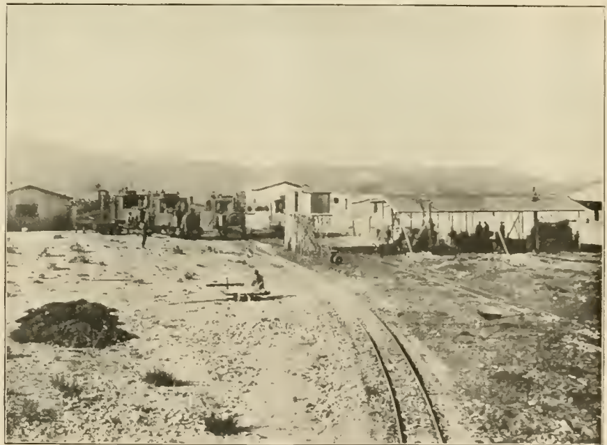
REPAIR SHOPS AT USAKOS, OTAVI RAILWAY.
